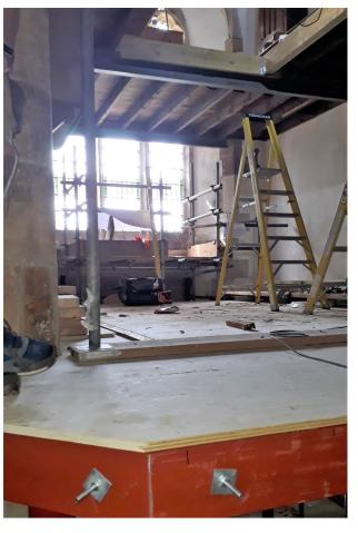
have taken the opportunity to make a provision for future removal of the bells by constructing "structural openings" in both the new mezzanine floor and the original bell ringing chamber floor above. These could be opened up in the future to allow the bells to be lowered from the belfry, but for now they are boarded over so nothing will be visible and there will be no risk of anyone falling through!
