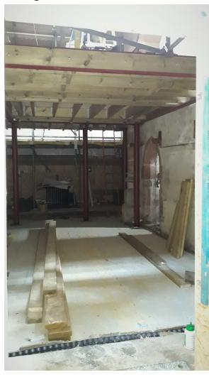
With the steel in place, the team of carpenters were able to build the new mezzanine floor. As part of the work we
